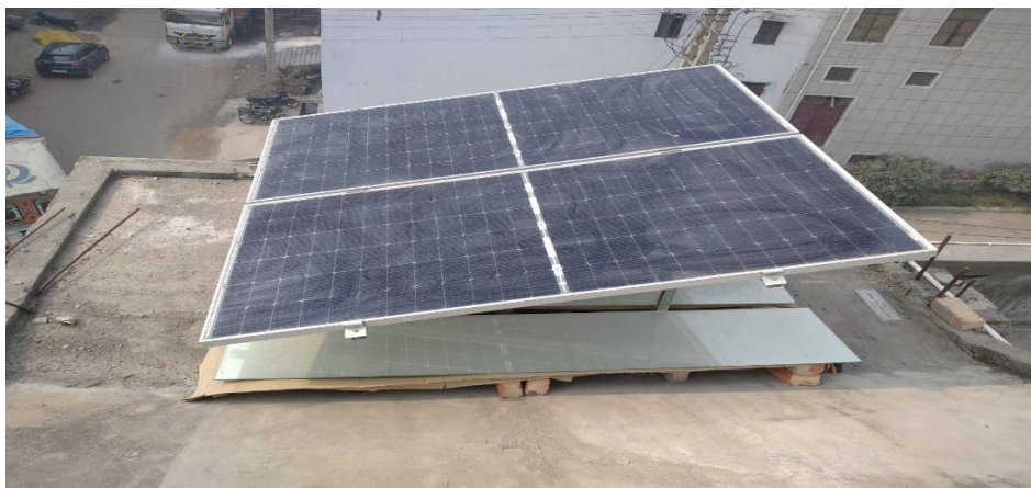
Figure 6. Mirror reflector with bi-facial PV module
