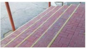
The following widths are required to prevent the disabled legs from slipping when moving. Materials 0.05 m - 0.065 m on steps and 0.03-0.055 m on the rise. Colored materials are recommended on the platforms.
