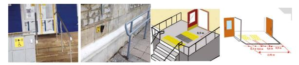
Outside the buildings, the width of the stairs should not be less than 1.35, which also means wheelchair access and fire times. At the height of the stairs, the height of each step is assumed not to exceed 12 cm. Proper projects are designed in the following order;
